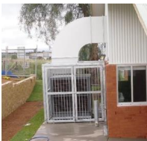
Figure 02: Air-conditioning plant enclosure
