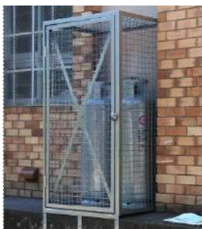
Figure 01: Gas tank enclosure
